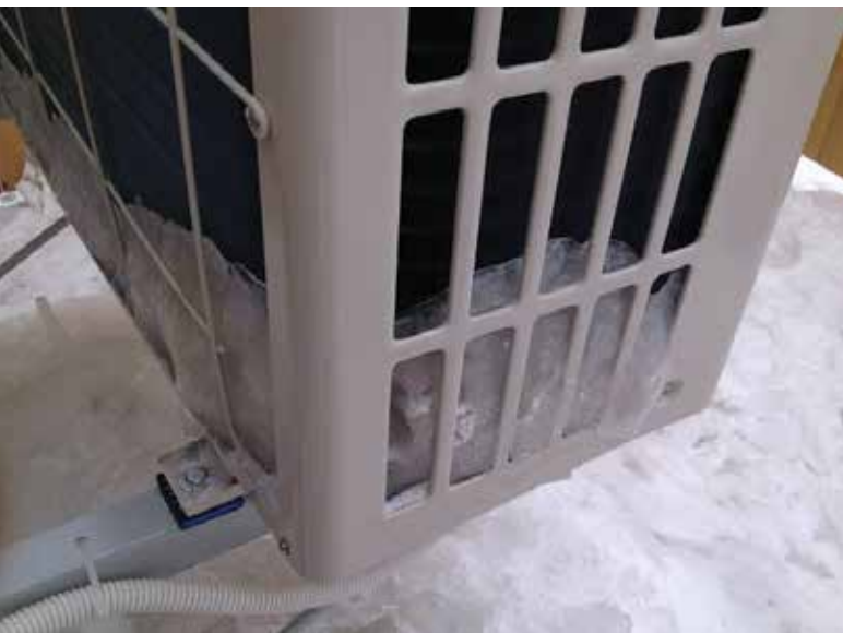
Without the right technology, condensate freezes in the bottom of the unit and reduces its efficiency and heating output.
